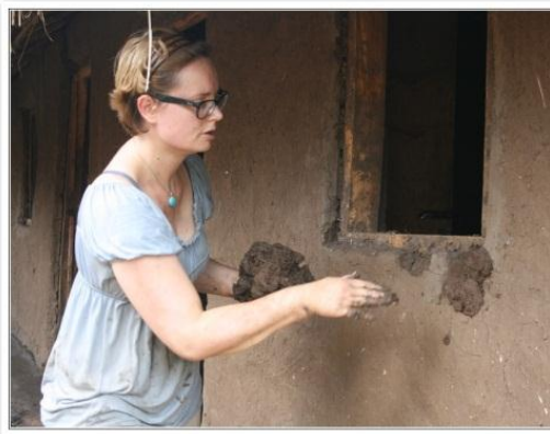
Iris repairing the walls (above)
