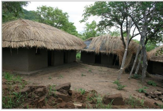
Before with new roofs
