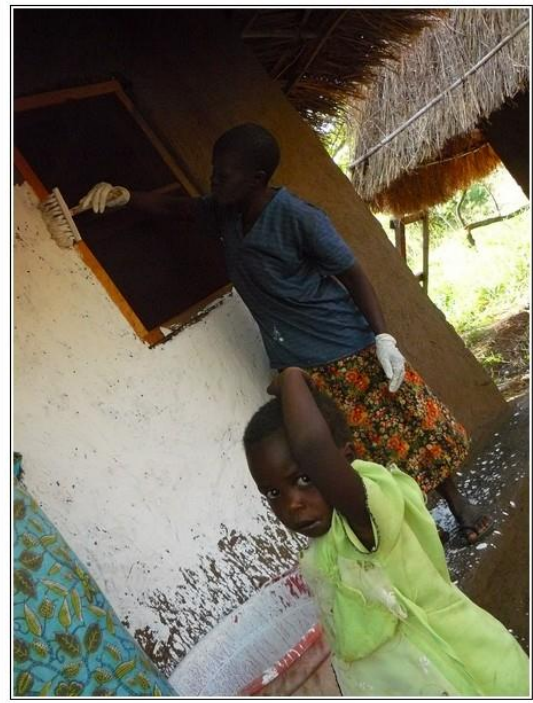
Painting the walls.
